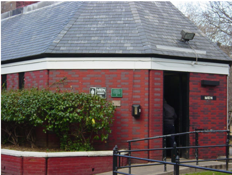
Fig. 4.3 Washington Square Park restroom
