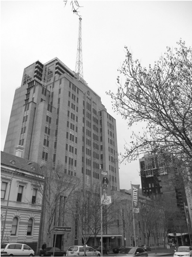
Figure 15.2 The Russell Street Police Headquarters and its striking Art Deco architectural style
